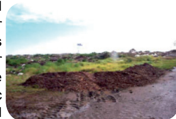
Freshly chipped RO formed into a berm
