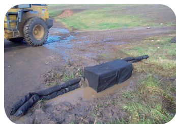
Installation of devices containing RO
