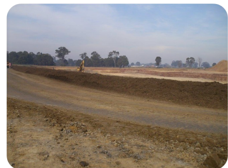
Epic Mines CoverAll™ application, NSW - Australia
