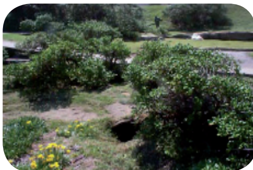
Exposed Drain prior to Enviro-media installation
