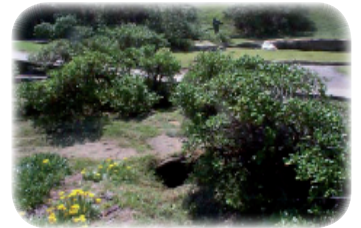
Exposed Drain prior to Enviro-media installation
