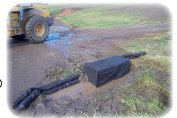
Installation of devices containing RO
